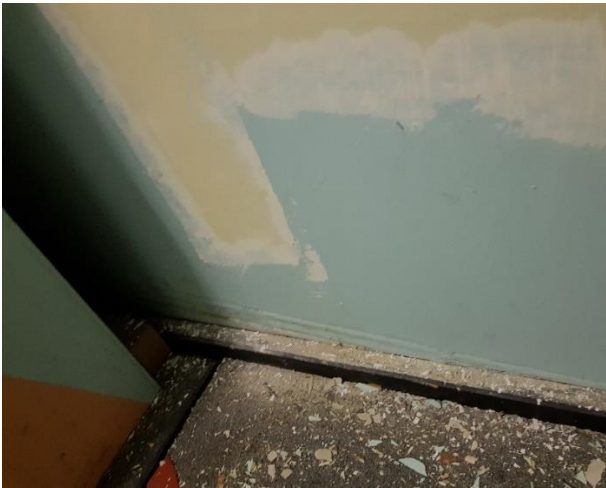
Figure 46 – Evidence of Dado line etched within the rendered plaster walling currently at floor level indicates a ramp existed previously at a lower level within this space
