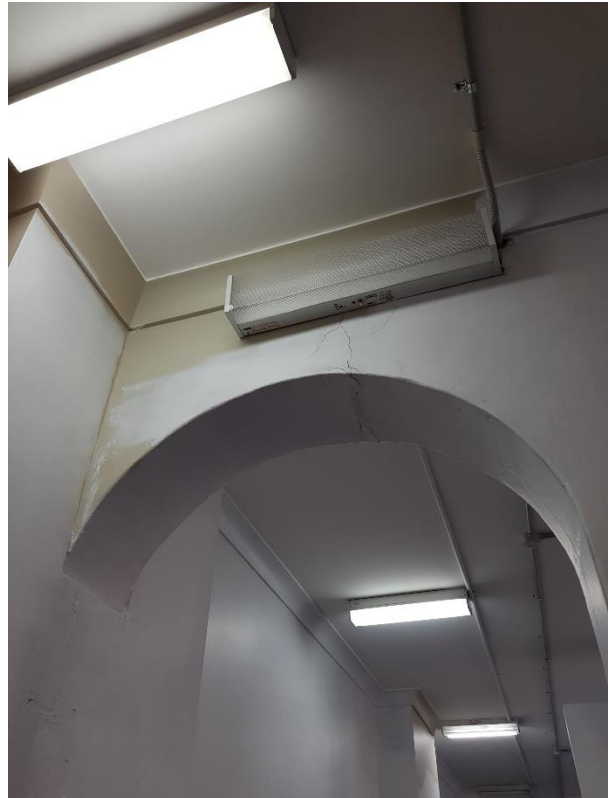
Figure 41 – First Floor, hall way showing arches abutting structural walls along the extent of the original masonry wall. Here the wall has a later addition plasterboard finish. Cracking is evident above the masonry arch.
