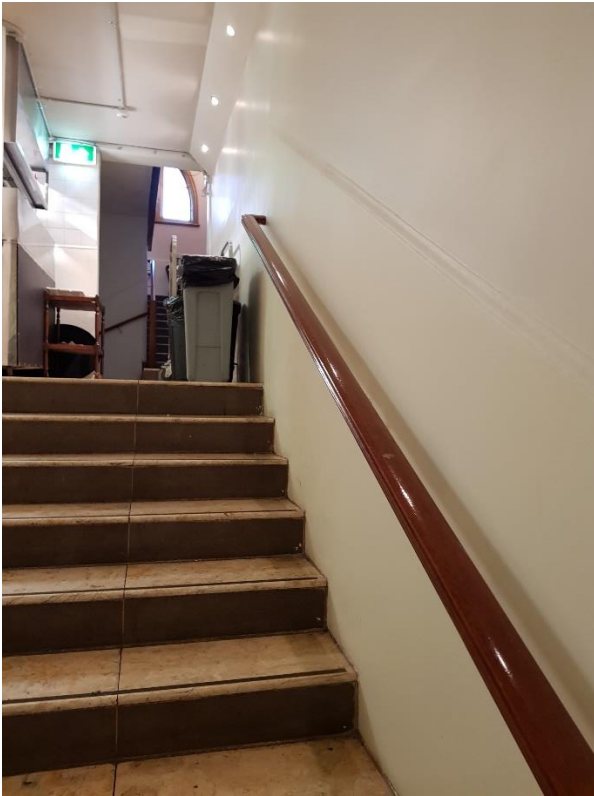
Figure 52 – Stairwell between Ground and Second Floors have rendered masonry walls. Stair tread and balustrading are later addition
