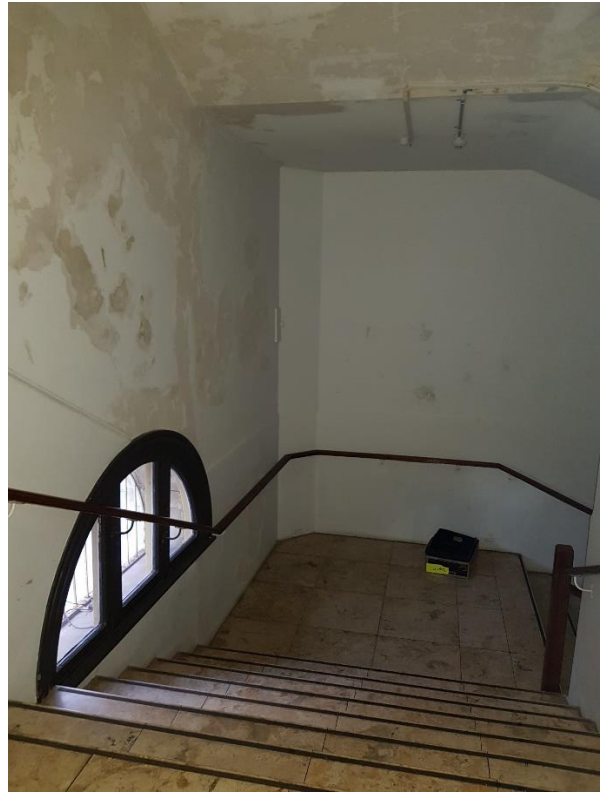
Figure 53 – Stairwell between Ground and Second Floors have rendered masonry walls. Stair tread and balustrading are later addition
