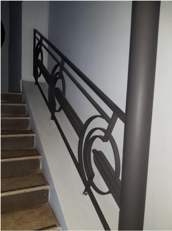
Figure 50 – Western stair with Art Deco inspired balustrading leading from Ground Floor entry foyer. The layout and finishes are later addition
