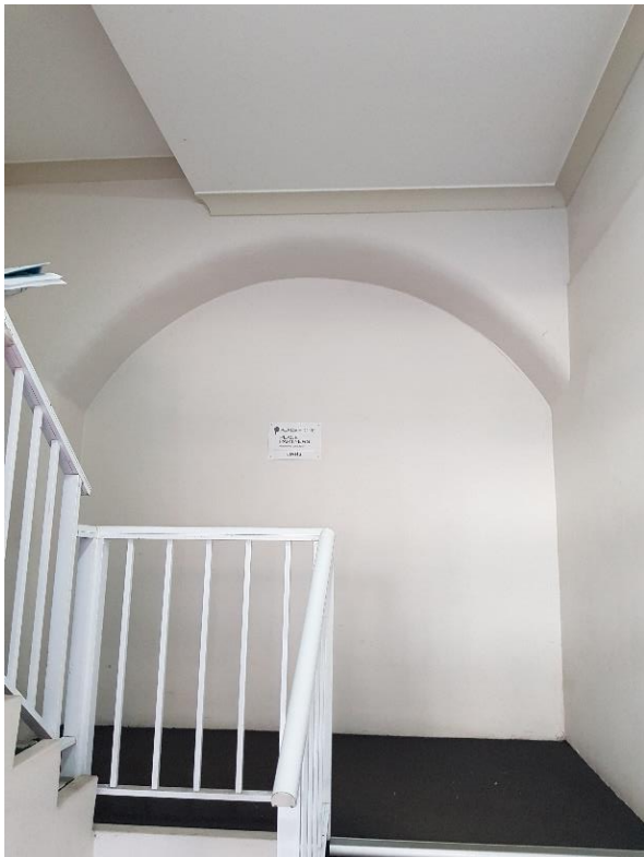
Figure 48 – Staircase between Ground and First Floors showing the recessed arch to the landing wall. Plaster board ceiling and cornices are later addition
