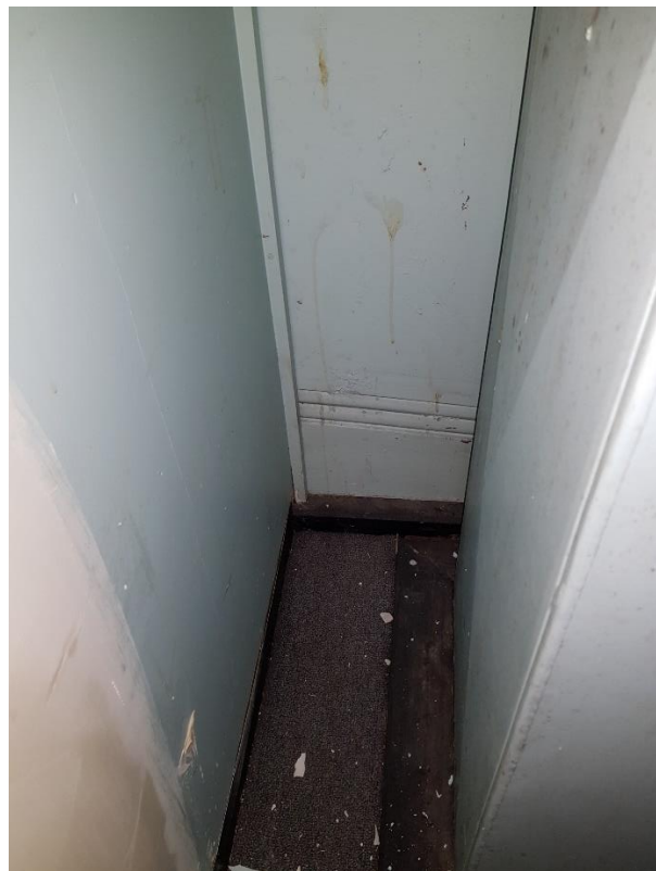
Figure 45 – Dado line etched within the rendered plaster walling indicates a ramp existed previously at a lower level within this space
